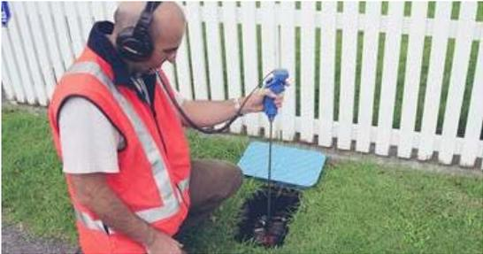
Above: acoustic technology used for leak detection
