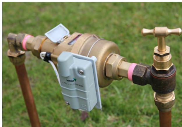
**Above:** The digital logger device attached to an existing customer water meter.
