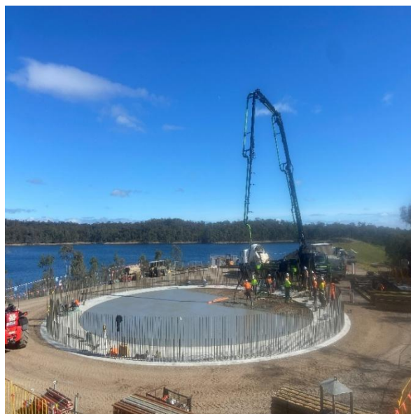
Construction of a 2 ML Class A recycled water storage at Spring Gully Reservoir
