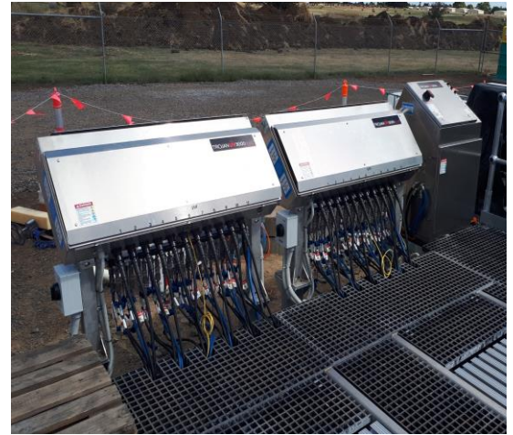
Above: New UV disinfection equipment installed
