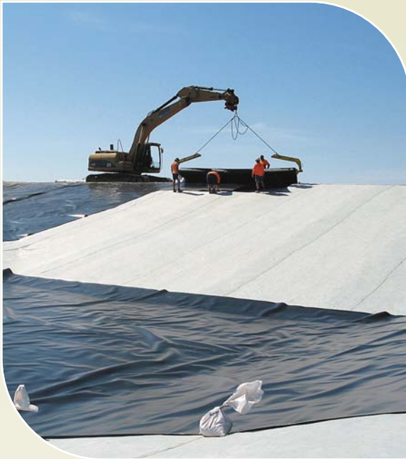
Storage lining at Korong Vale, November 2009
