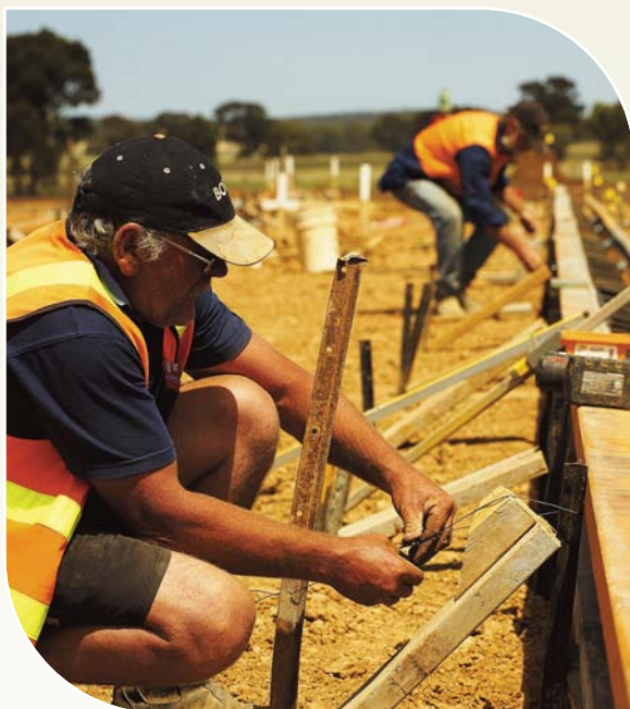
Construction at the Korong Vale basins, November 2009
