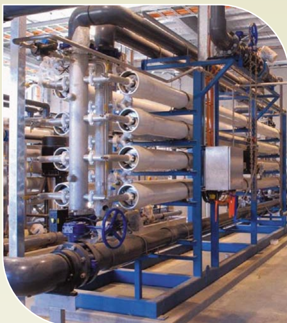
Bendigo Recycled Water Factory
