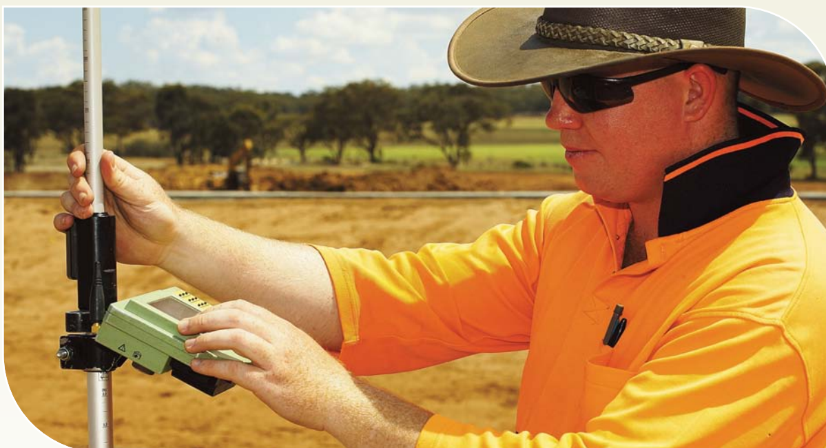
Construction at the Korong Vale basins, November 2009
