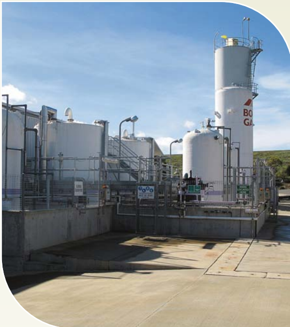
Bendigo Water Treatment Plant
