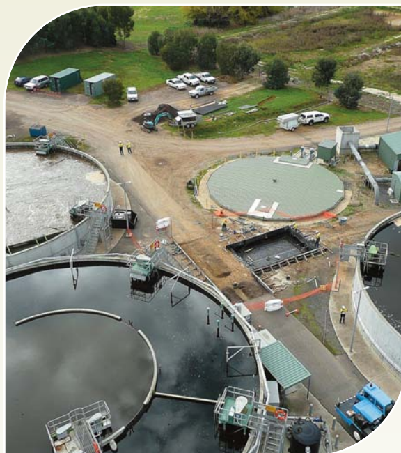
Castlemaine Water Reclamation Plant
