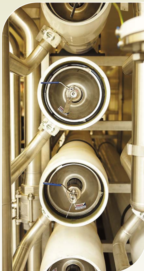
Reverse Osmosis membranes, Bridgewater Desalination Plant, November 2009
