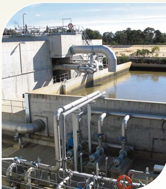
Bendigo Water Treatment Plant
